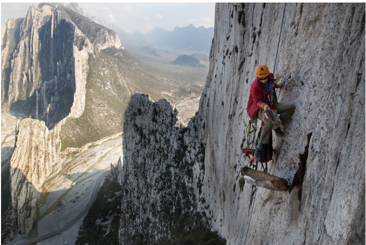
Gareth Leah cleaning a loose block on the Life You Can Save (350m, 13 pitches, 5.12d).
