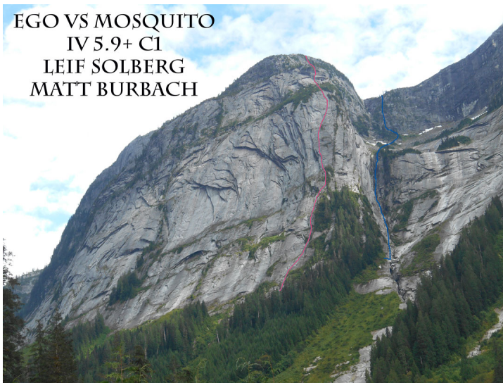
The route line for Ego vs. Mosquito (900m, 5.9+ C1) on the north face of the Penguin. Ascent line in red, descent in blue. This formation is just to the east of the larger Super Unknown wall.
