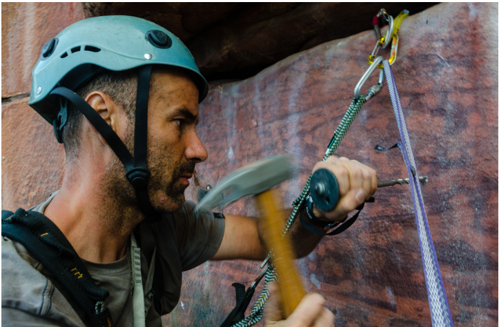
Drilling a belay anchor.
